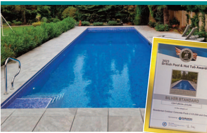
2023 SPATA SILVER AWARD Concrete Pool. Another fine example of traditionally built pool on the Essex/Hertford borders.
